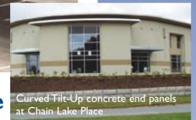
Curved Tilt-Up concrete end panels at Chain Lake Place
