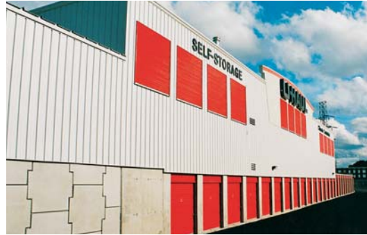
The new U-Haul Co. Ltd. building in Dartmouth was a challenge to build on the steep, rocky site.
